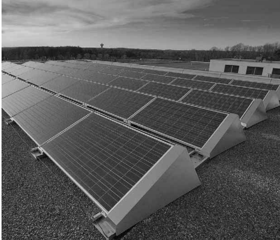
Powering education: Ontario schools range from 750 sf to 270,000 sf and school boards are facing a variety of energy challenges.
